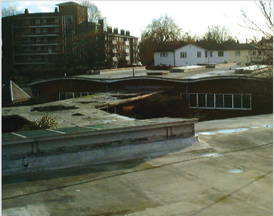
Before refurbishment: The roof had been patch repaired on numerous occasions to try and extend the life of the existing waterproofing, but even these were starting to fail (See front for 'after' photograph).
